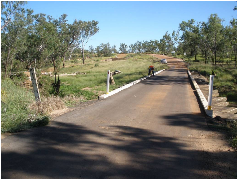
Figure 3-7 Clermont-Alpha Road - Narrow and Sealed Floodway Crossing
