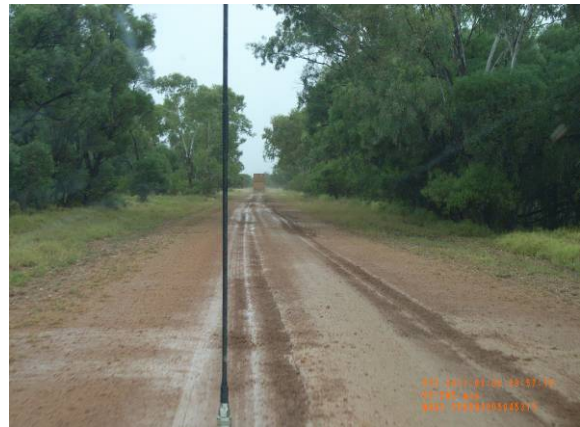
Light gravel over sandy base after rain and one road train
